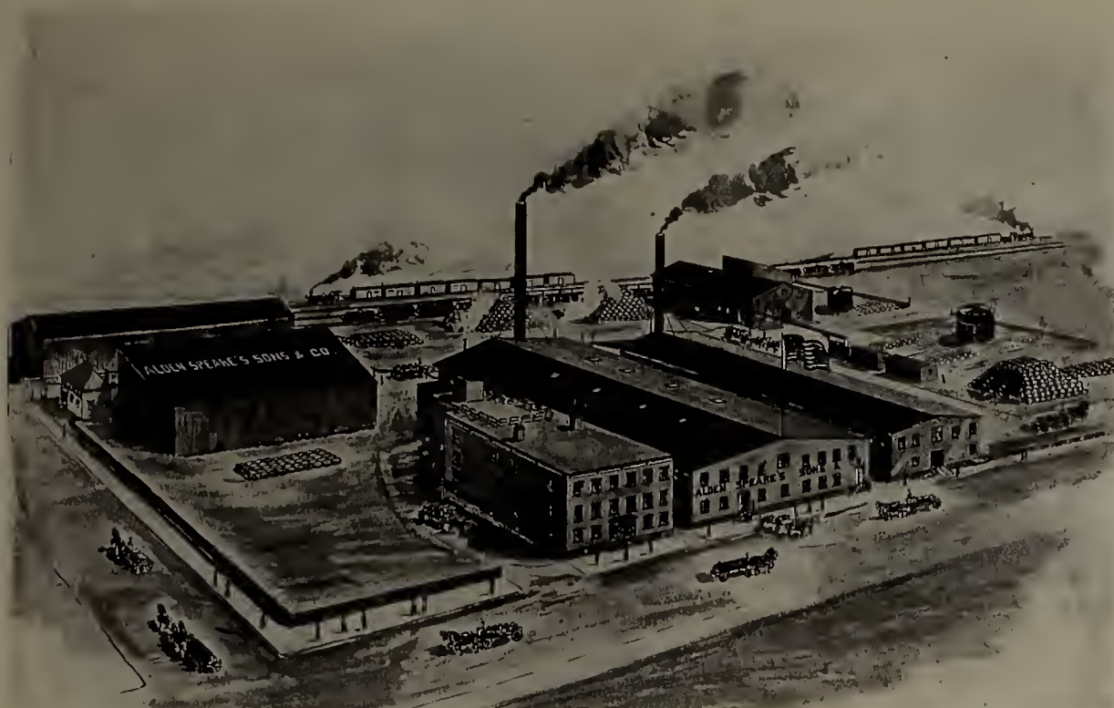
WORKS OF ALDEN SPEARE'S SONS & CO., Oil, Starch, and General Mill Supplies, East Cambridge, Mass.
